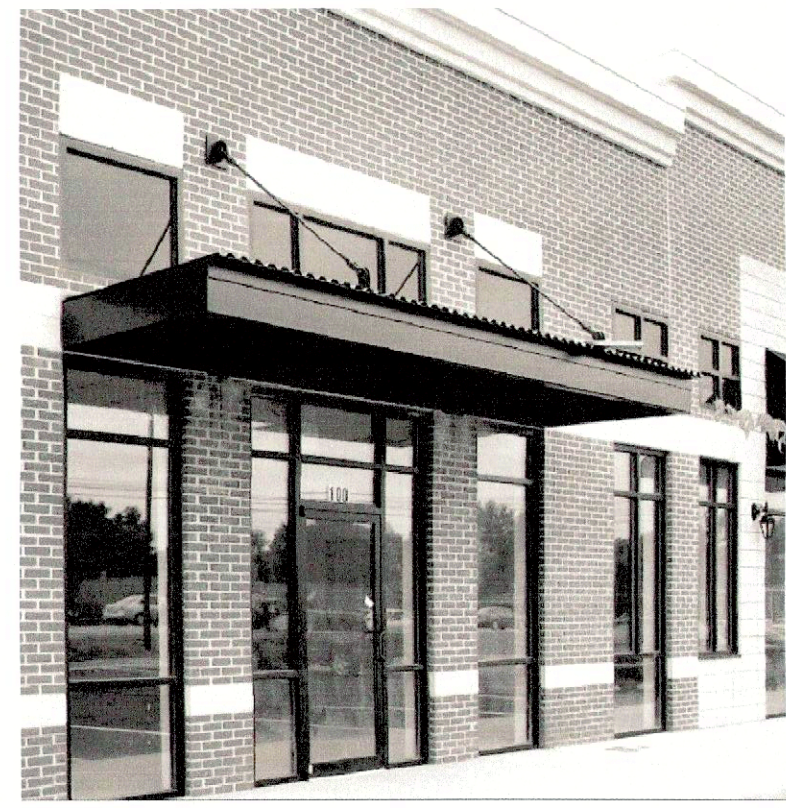
DARK BRONZE FRAMES, PARAPET CAP & CANOPY
