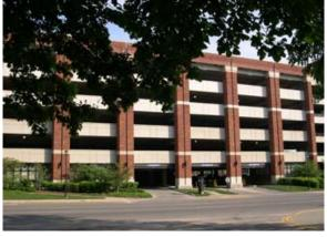
Precast Spandrel Panels With Enhanced Detailing Required
