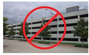
Precast Spandrel Panels With No Detailing Are Not Permitted
