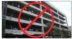
Exposed Slab and Cable Guard Rails Are Not Permitted
