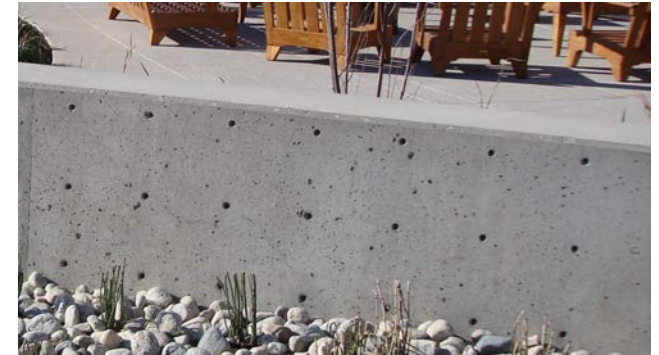
FORM FINISHED CONCRETE WALL W/ EXPOSED TIE-BACK PATTERN
