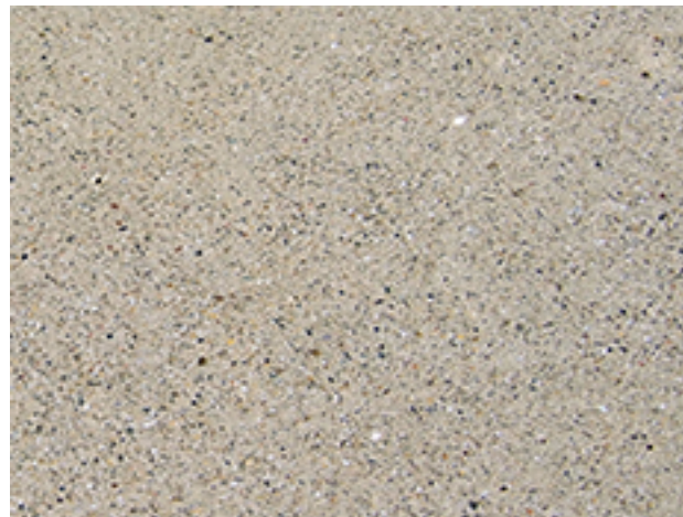
CAST STONE WINDOW SILL, BUILDING BASE
