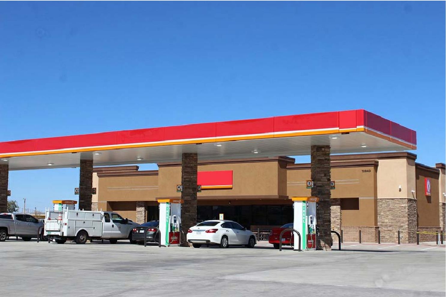
BUILDING COLOR AND MATERIAL SAMPLE
