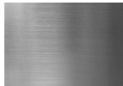
Galvanized Metal Awning / Eyebrow
