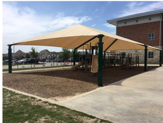
NOTE: PROVIDE A MINIMUM OF 10'-0" CLEARANCE UNDER THE LOWEST PORTION OF THE SHADE STRUCTURE - THE ACTUAL HEIGHT OF THE SHADE STRUCTURE TO BE COORDINATED WITH THE OWNER'S PLAYGROUND VENDOR TO ENSURE MINIMUM CLEARANCES ARE HELD.
