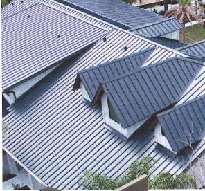
The Berridge Cee-Lock Panel is an architectural metal standing seam panel that incorporates an integral snap-lock seam and an optional patented vinyl weatherseal.
