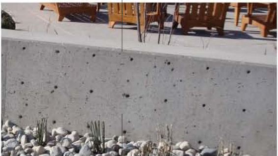
Form Finished Concrete Retaining Wall With Exposed Tie-Back Pattern
