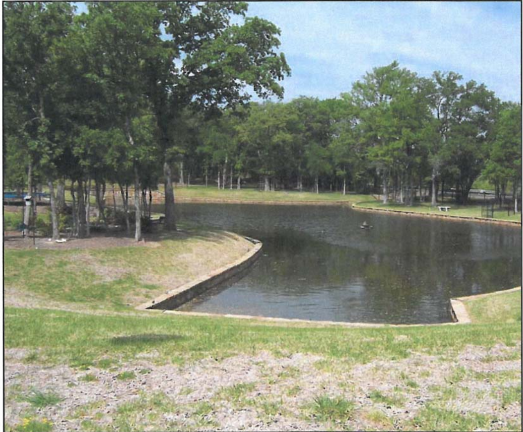
Figure 5: Retention Pond with Hardedge.
