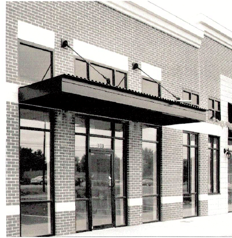
DARK BRONZE FRAMES, PARAPET CAP & CANOPY
